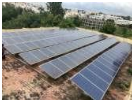
ROOF TOP SOLAR SYSTEM 160 KWp
