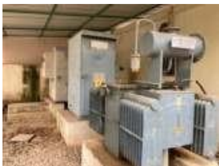
TRANSFORMER RATING 200 KVA
